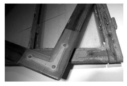
*Figure 1* Windows from 1880, showing small-scale repairs.
